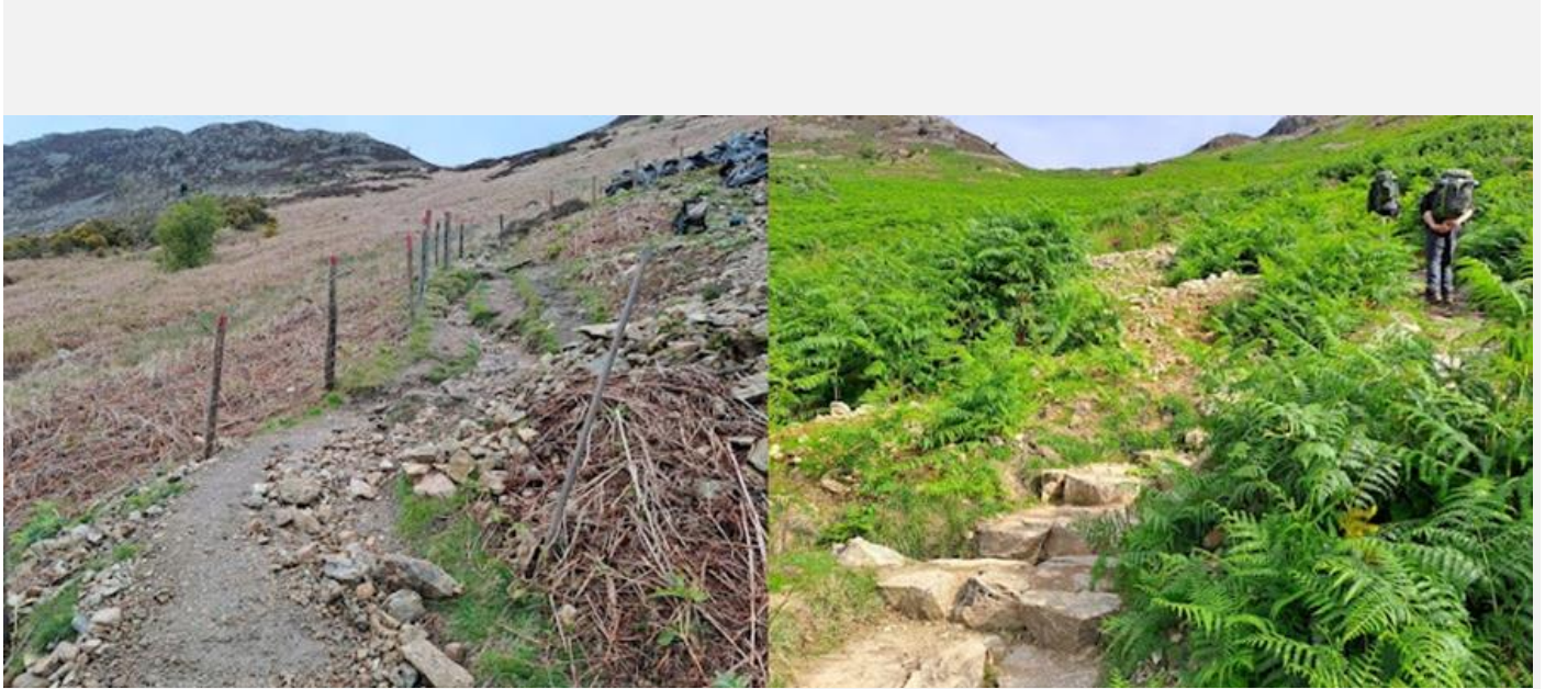
Photos: Before work started on Glenridding Dodd
